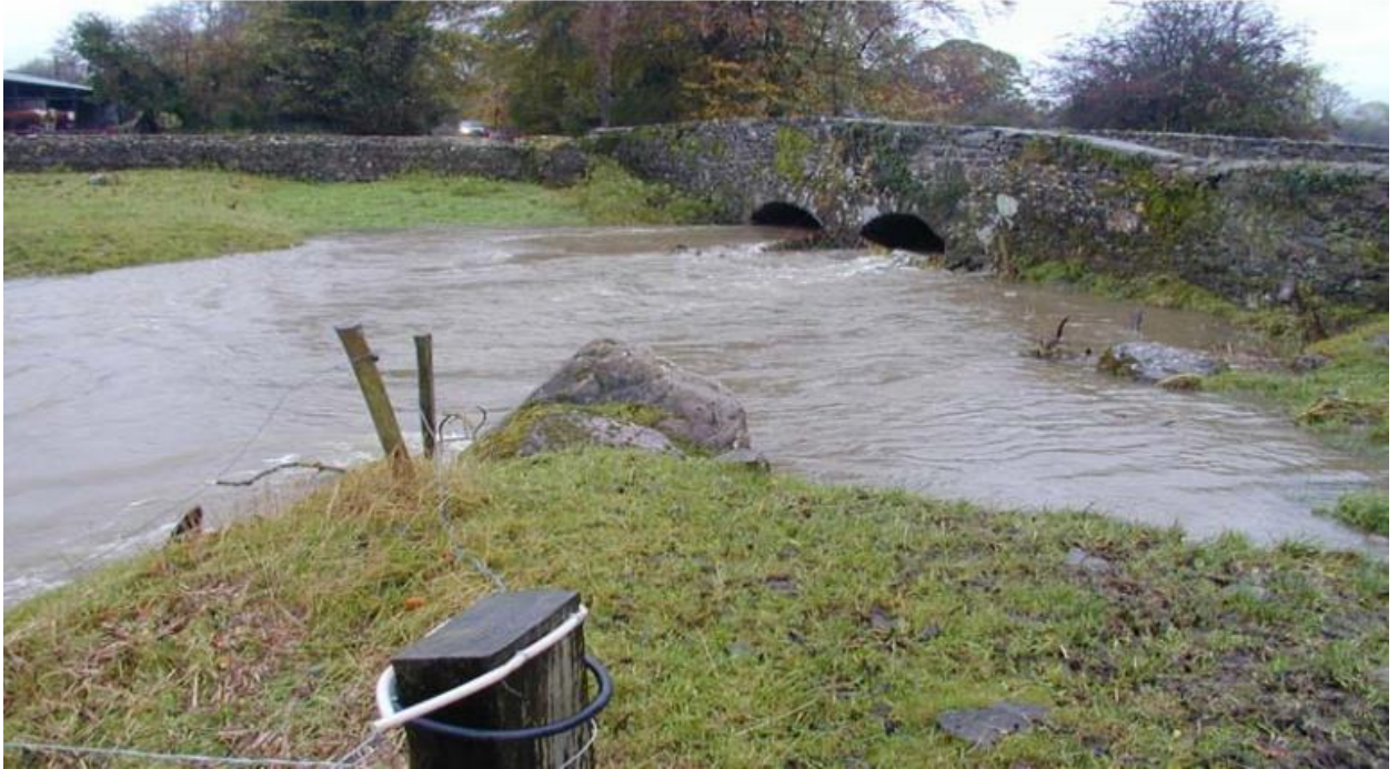
Figure 5a - Downstream of Painestown Bridge during Flooding (8 th November 2000)
